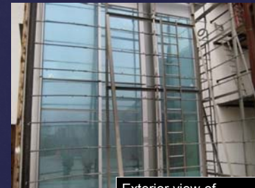
Exterior view of chamber under seismic loading of 1.4" lateral
