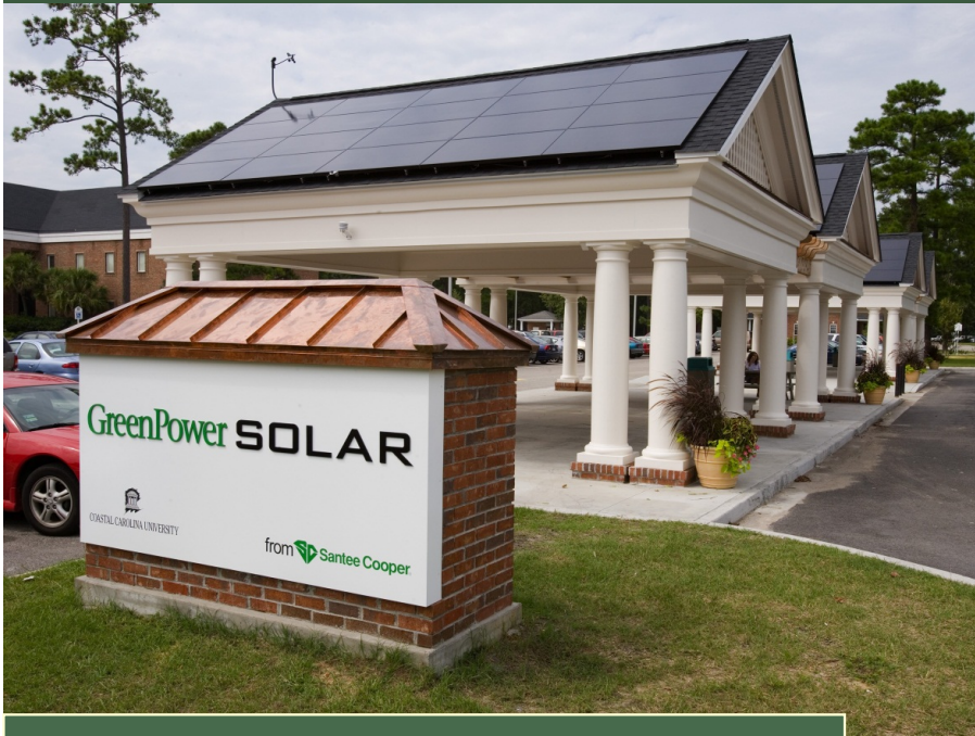
Solar Pavilions at Coastal Carolina University
