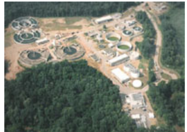
Mauldin Road WWTP
