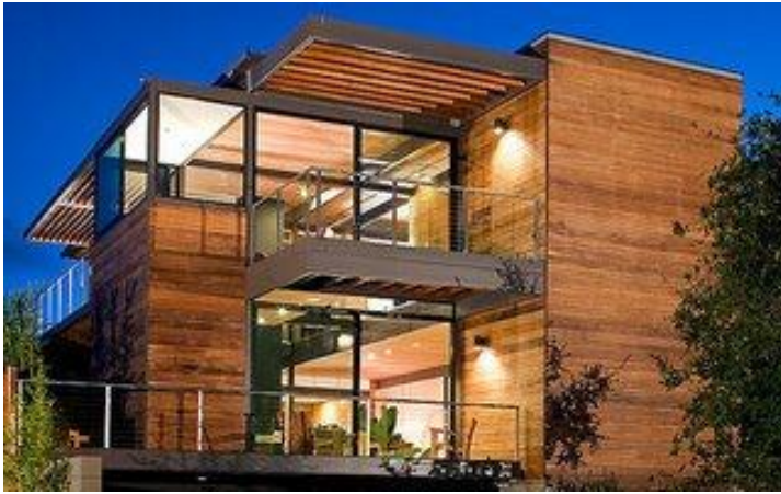
Steve Glenn's Santa Monica house, first house platinum LEED
