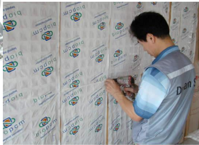
Biopcm™ layered on top of insulation in a standard wood frame structure.
