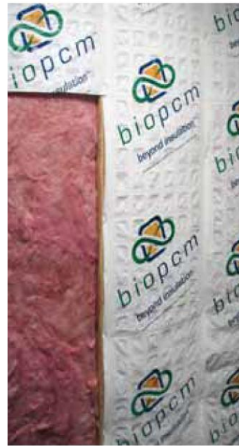
Biopcm™ layered on top of insulation in a standard wood frame structure.
