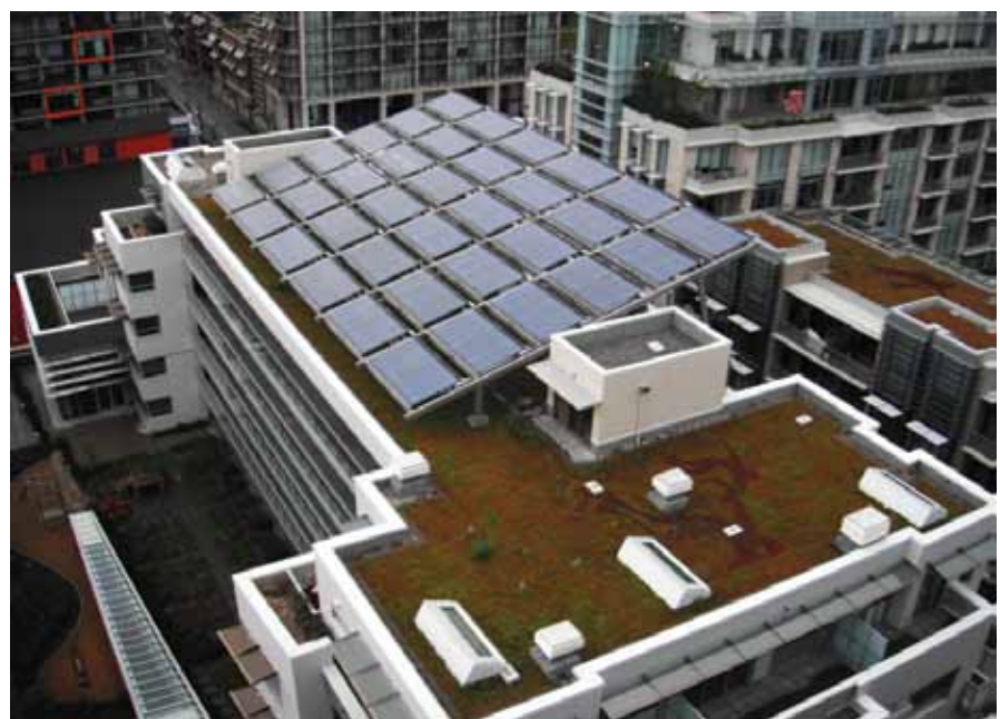
Figure 3. Green roof with solar hot water heating panels; a net-zero building.
