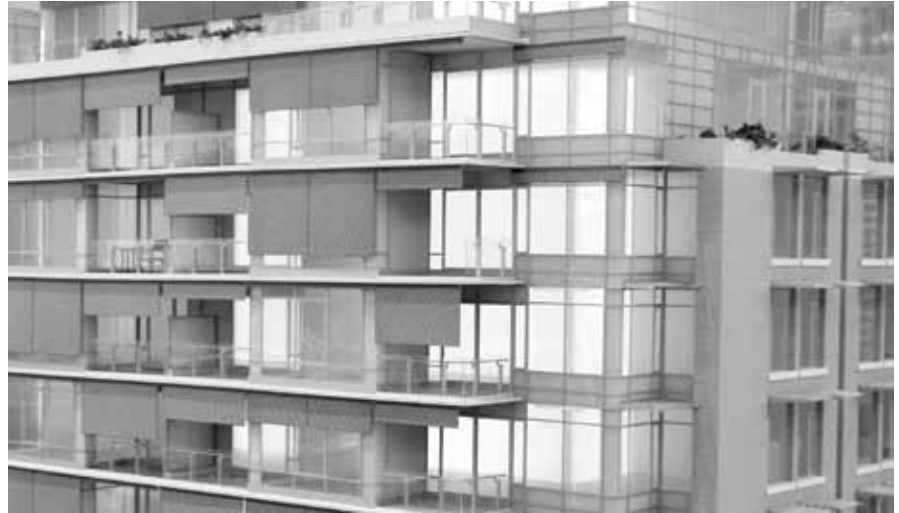
Figure 1. The shading strategy included automated vertical shades on the west façade (left) and horizontal shades on the southern elevation (right).
